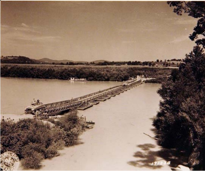
Sherman tanks cross 600-foot long pontoon bridge near Rome in Smith County, Aug. 14, 1943.
